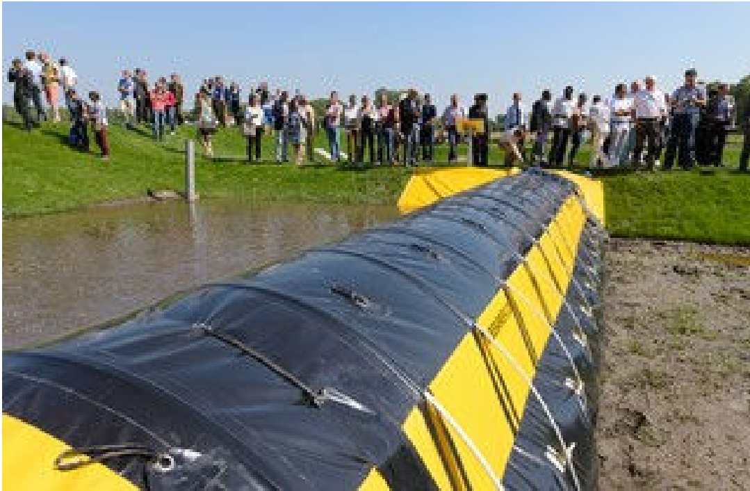
Figure 6 Tube Barrier, an innovative concept to fight floods with water (courtesy.tubebarrier.com)
