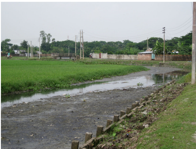
Figure 5 Reduction in discharge capacity due to lack of maintenance in Khulna, Bangladesh
