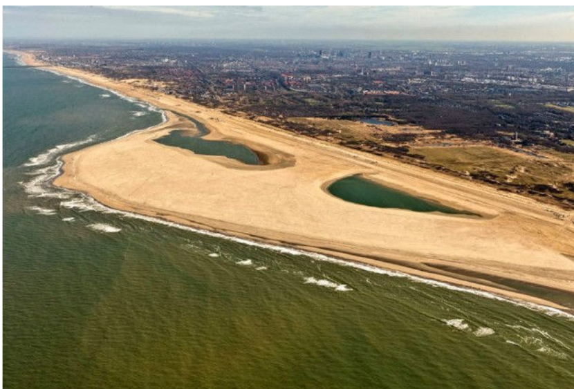
Figure 7 Formation of a sand supplied barrier in front of the Dutch coast
